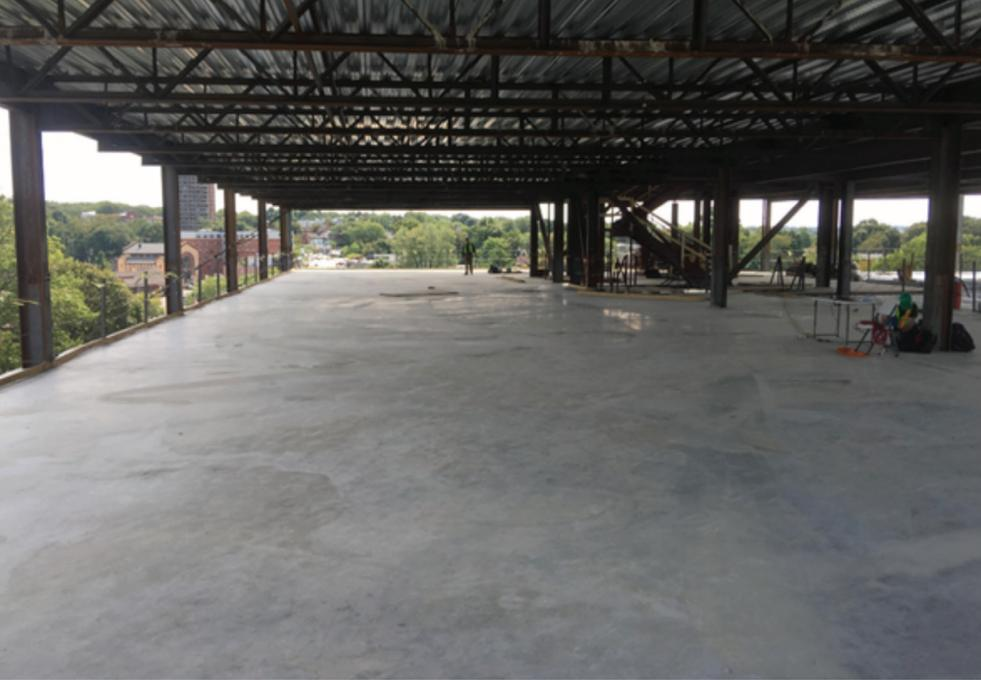
Figure 7 View of Tested Floor Having Flush Frame Joist Connections.
