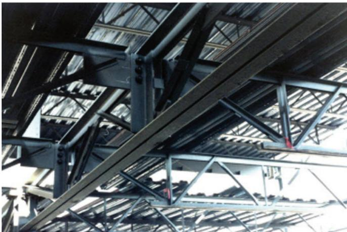
Figure 2 Flush Frame Joist End Connections.
